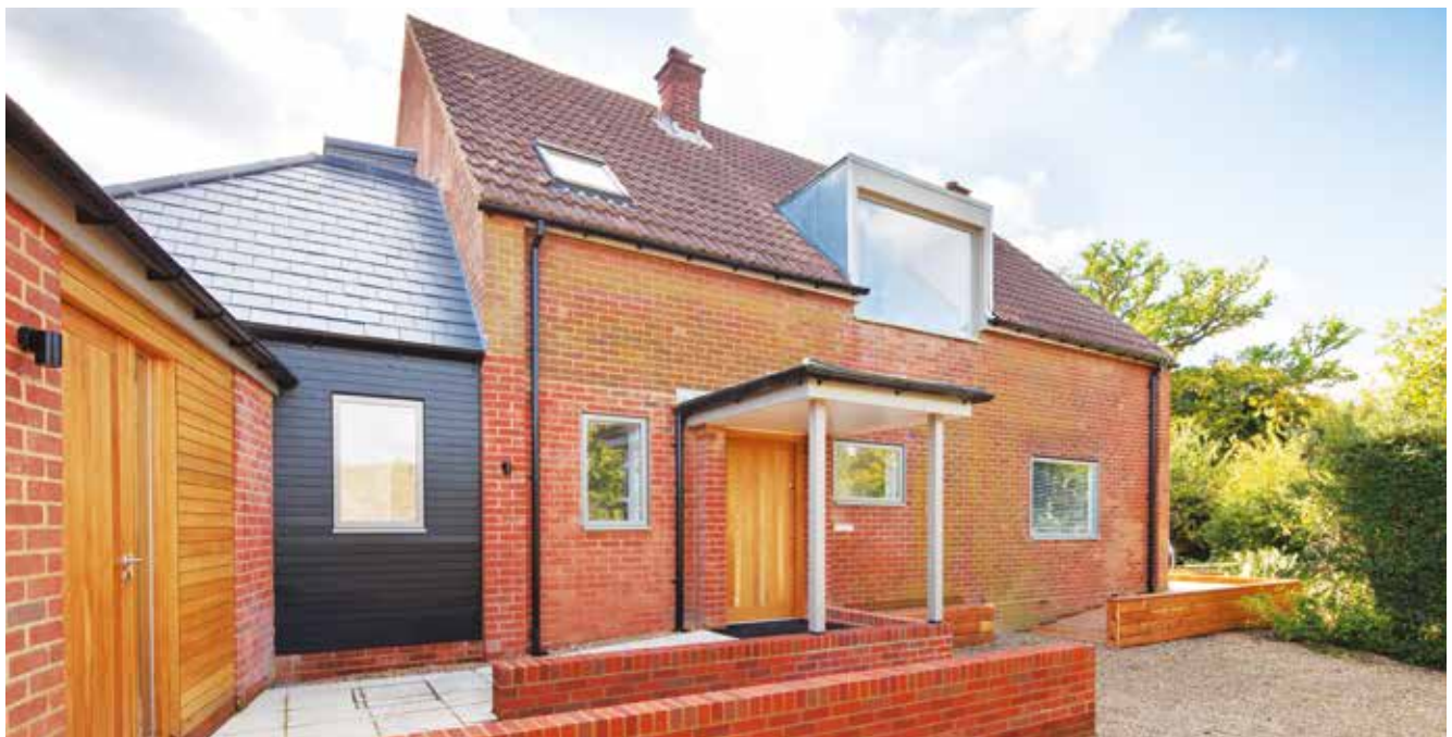
Making the decking flush with the house allows Joseph to access the garden in his wheelchair
